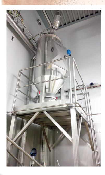
Our dust-extraction filters consist of a steel plate frame, cover and collection tank. The cover has a centrifuge vacuum, which generates a vacuum inside the vacuum tank and pipes. A control unit and compressed air tank are mounted to the filter frame.
