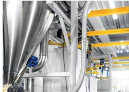
units to weighing hopper by vacuum conveyors. A major benefit is the completely dust-free conveying of material.
